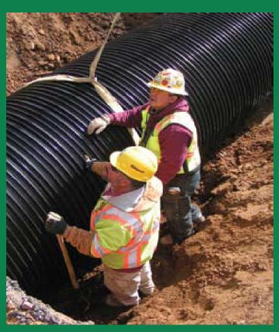
New material specification that allows the use of steel reinforced HDPE in liner applications.
